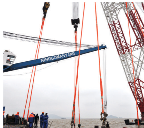
超高分子量聚乙烯缆绳应用于重型起吊 The HMPE rope applies to heavy lifting
